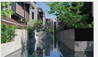
Watten Residences Strata Houses, Singapore SIA Architectural Design Award 2012
